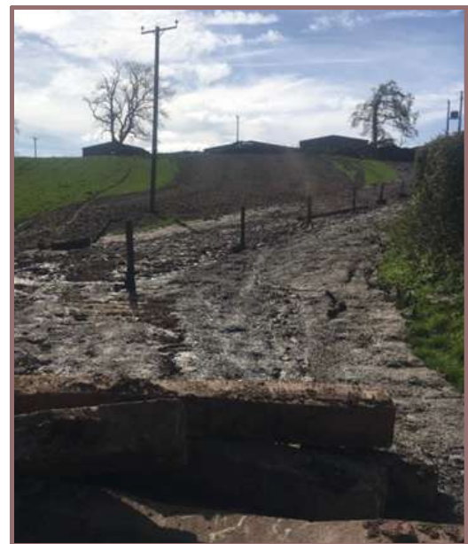
A section of concrete wall forming a slurry store failed leading to a loss of approximately 500,000 litres of cattle slurry © Oracle Environmental Experts
