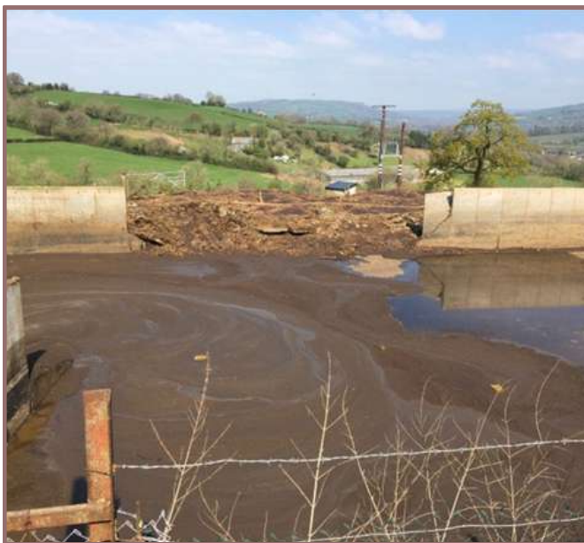
A section of concrete wall forming a slurry store failed leading to a loss of approximately 500,000 litres of cattle slurry © Oracle Environmental Experts
